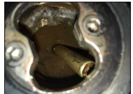
Brass tubing insert installed.
